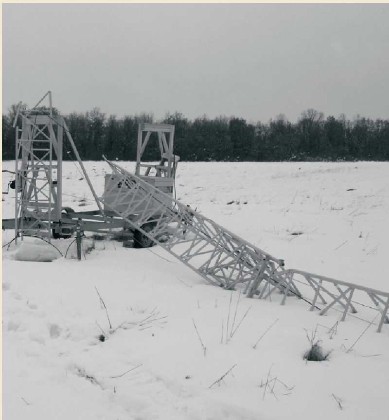
Heavy snow downed a portable tower which supported radio communications for the County 27 Fire near Karlstad. Photo by Kevin Throop, USFS, Superior National Forest
