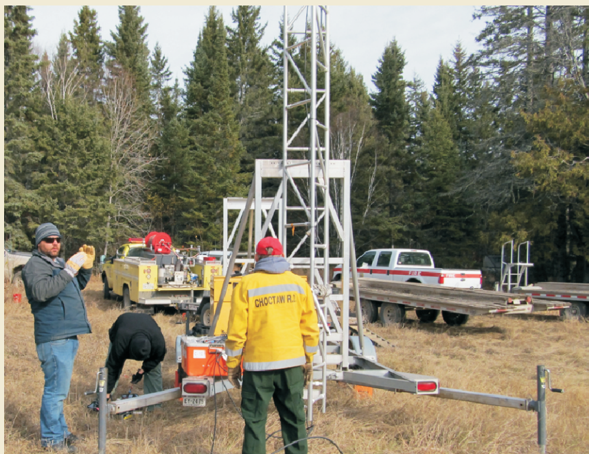
Team members install a portable repeater tower on the North Minnie Fire. Photo by Dana Carlson, DNR, Baudette
