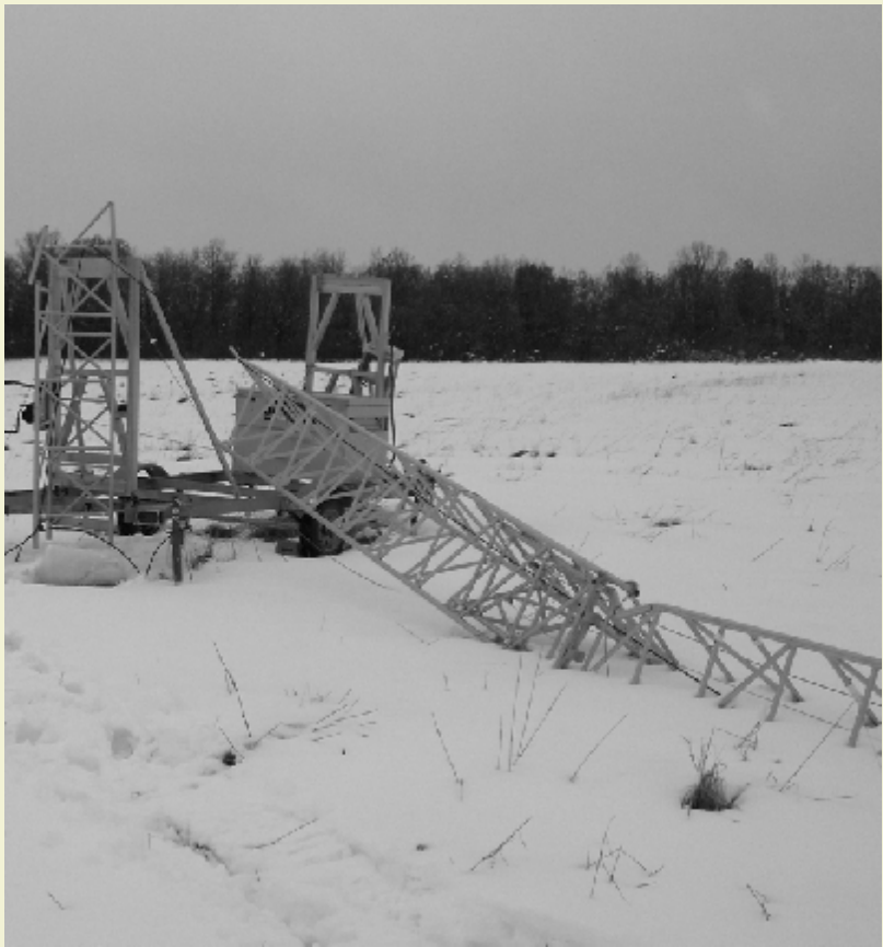
Heavy snow downed a portable tower which supported radio communications for the County 27 Fire near Karlstad. Photo by Kevin Throop, USFS, Superior National Forest
