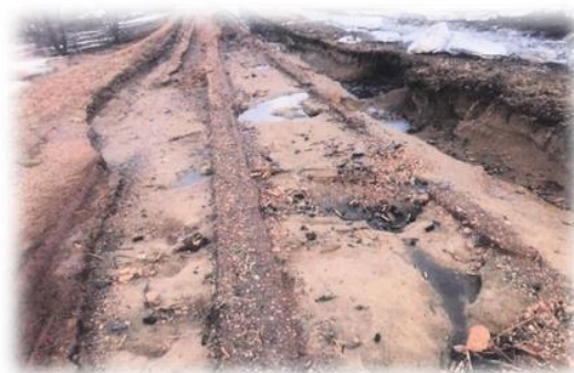
Figure 4: Road washout due to spring flooding, photo credit: DPS
